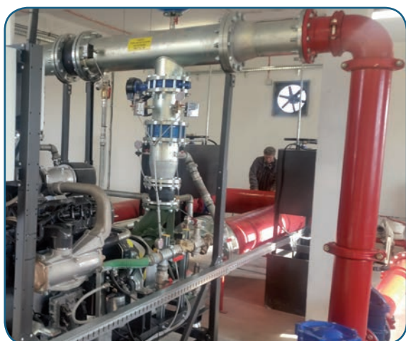
Motopompa tipo "vertical turbine pump" insonorizzata, realizzata secondo UNI EN 12845 Soundproof Fire fighting Diesel motor pump with "vertical turbine pump", made according to standard EN 12845 Motobomba Diesel contra incendio insonorizada con "vertical turbine pump", realizada en acuerdo de EN 12845
