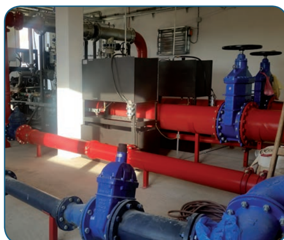
Motopompa tipo "vertical turbine pump" insonorizzata, realizzata secondo UNI EN 12845 Soundproof Fire fighting Diesel motor pump with "vertical turbine pump", made according to standard EN 12845 Motobomba Diesel contra incendio insonorizada con "vertical turbine pump", realizada en acuerdo de EN 12845
